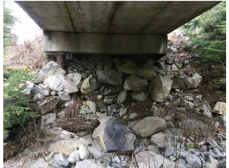
Right Bank Abutment when facing downstream
