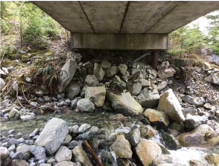
Left Bank Abutment when facing downstream
